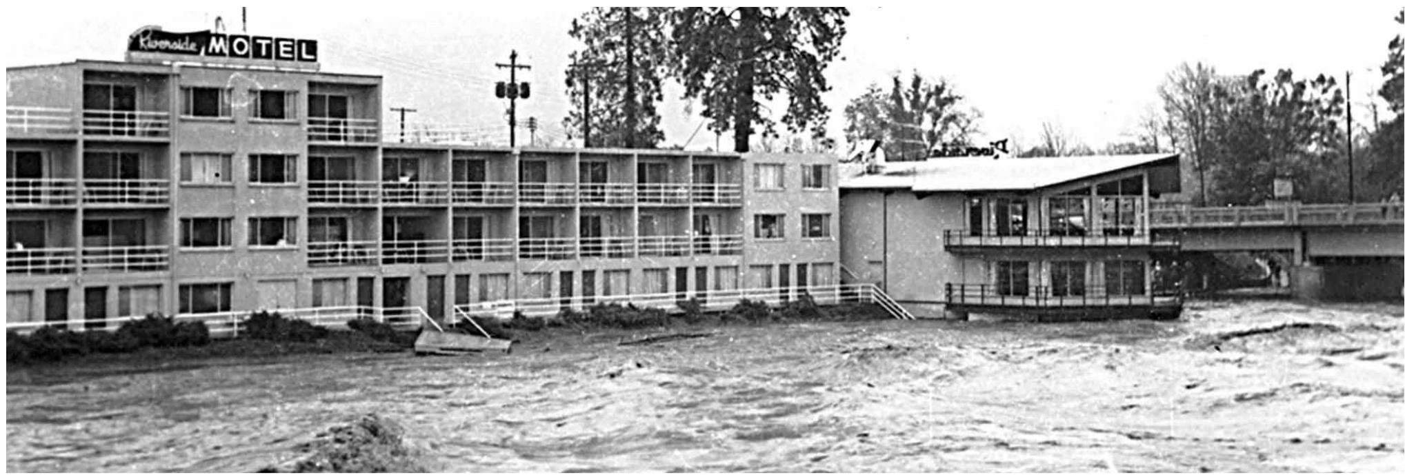
The Riverside Motel was swamped during the 1964 flood, when the Rogue River peaked 14.5 feet above flood stage the morning of Dec. 23. Huge swaths of the Rogue, Applegate and Illinois river valleys were stinking mud pits in the aftermath.
