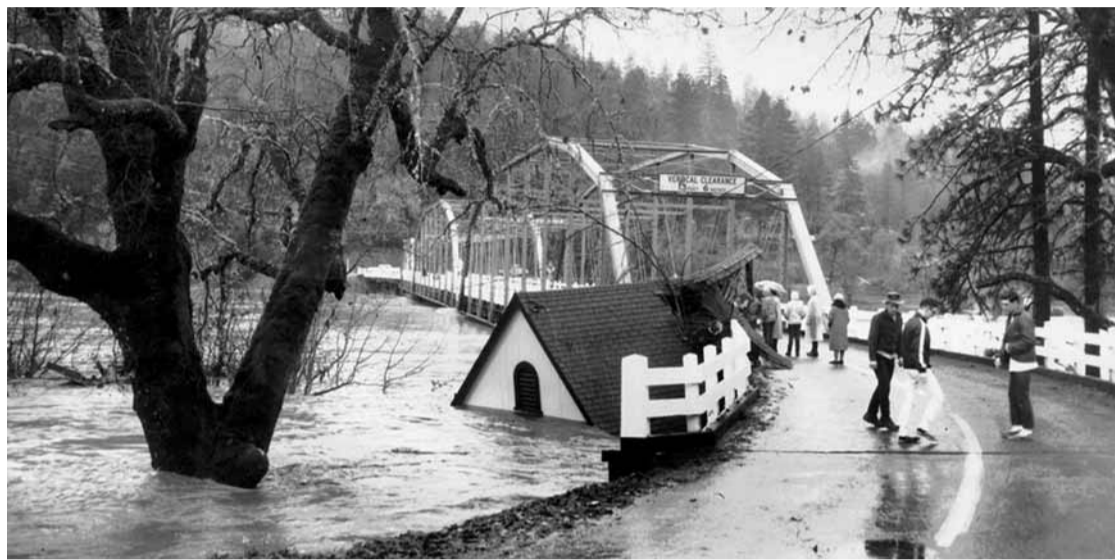
A house is hung up on Robertson Bridge in the flood of 1964 as Grants Pass High School students survey the damage.
